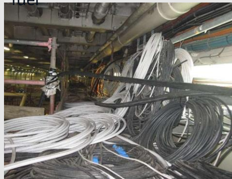
New electrical installation
