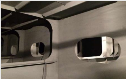
Methanol storage tank painted with zinc silicate
